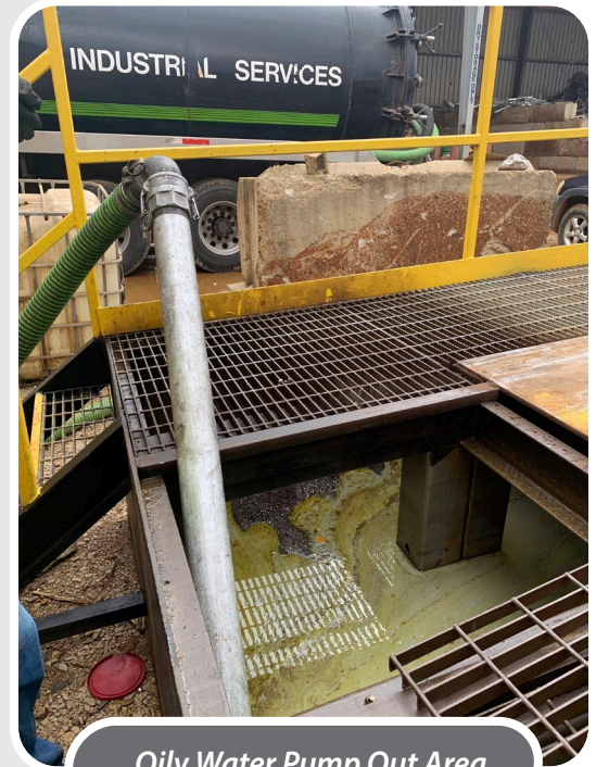
Oily Water Pump Out Area
