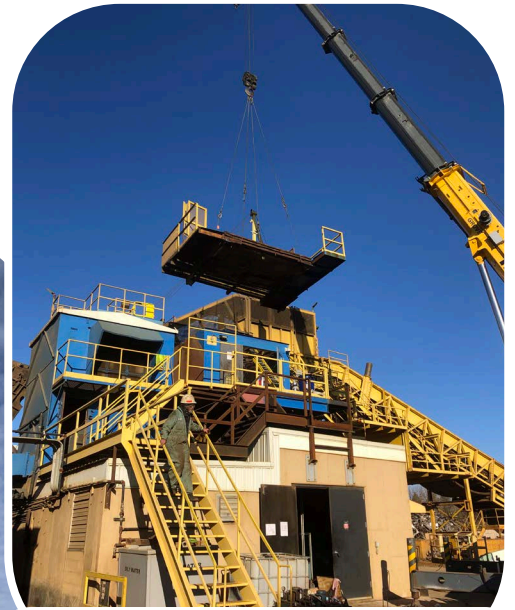
Old Shredder Deck Removal
