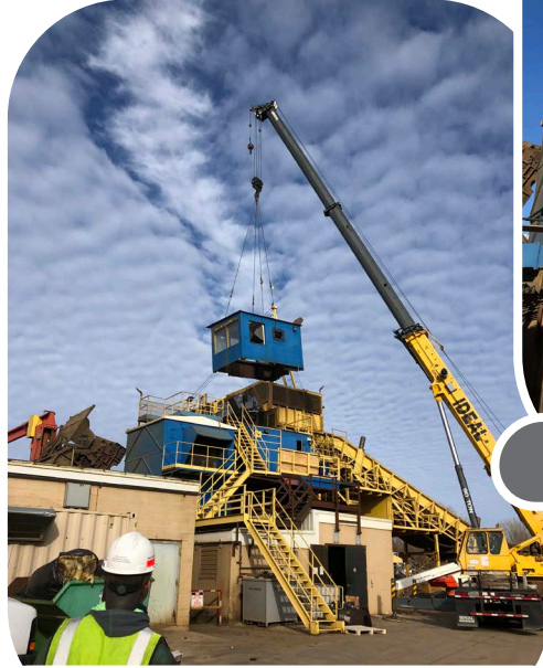
Old Shredder Cab Removal
