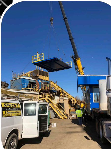
New Shredder Deck Lift
